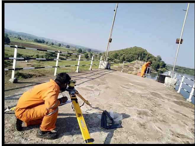
Level transfer from Fuse Gate to OBS CHOPADVAV
