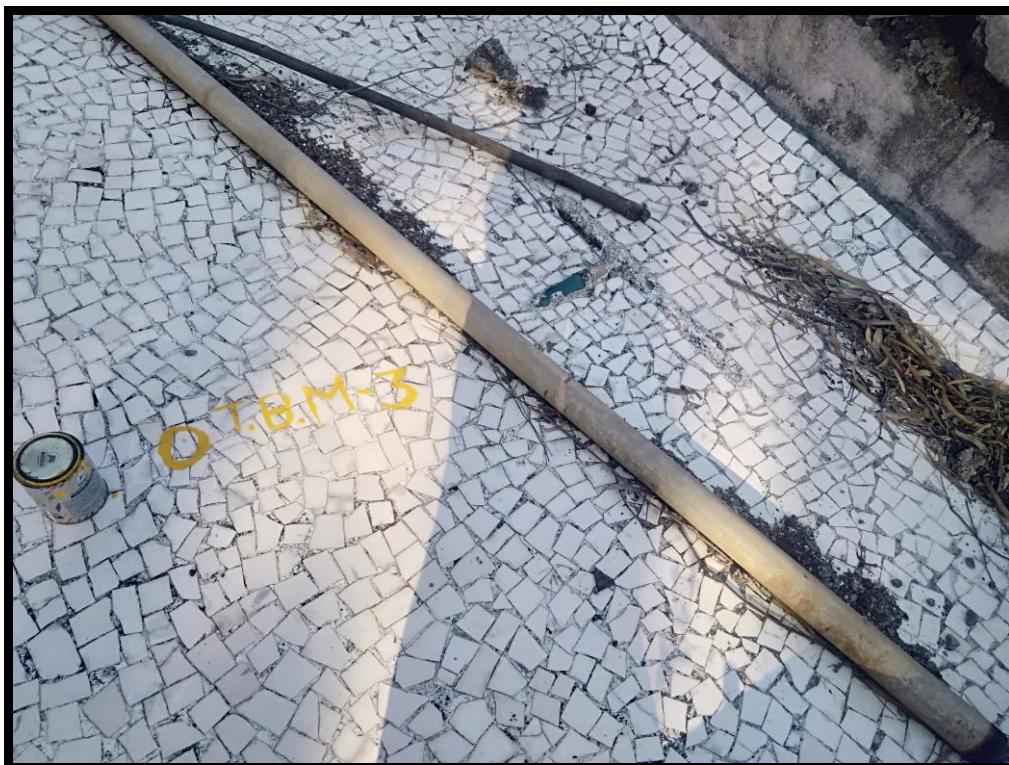
TBM 3 on Dam Guesthouse Top
